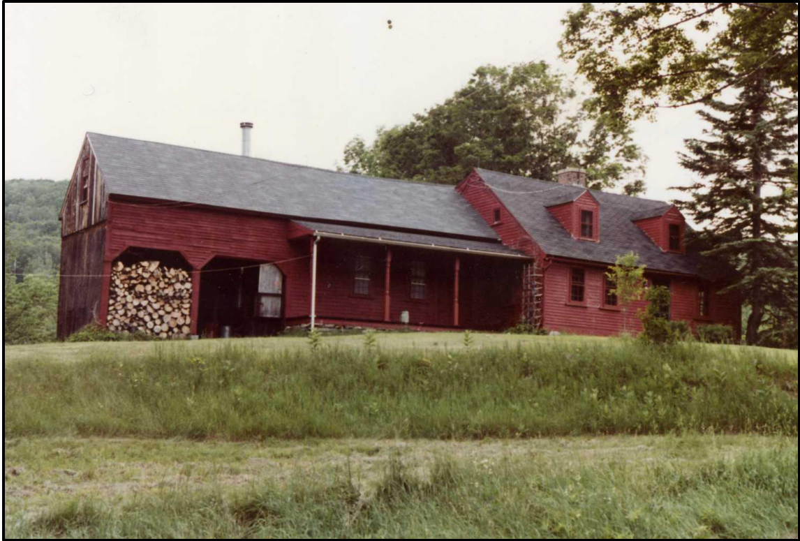
After many months, a frame house was completed. (1981 photo)
